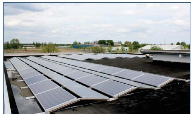
Fig. 1 Photovoltaic system installed on the roof of Allresist
